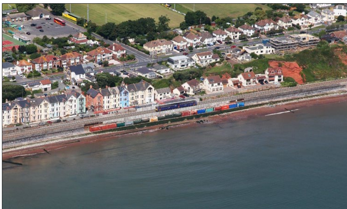
Figure 1.1: Emergency Repairs on Dawlish Seawall. Photograph provided with permission from Metcalfe (2015).
