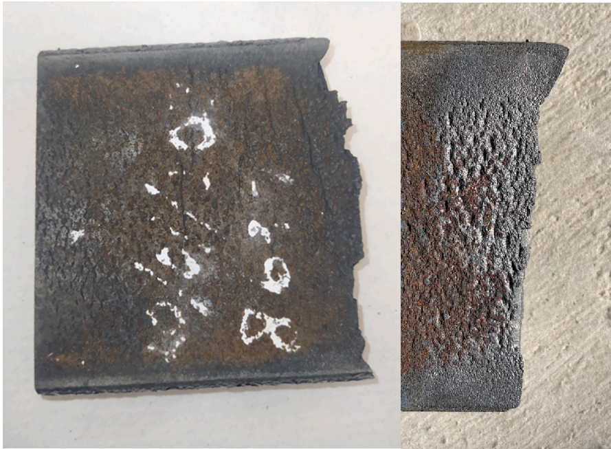
Fig. 4b. A colony of surface cracks can be seen on the tension surface, running parallel with the fracture surface. The image shows two different fracture surfaces and the one on the right has been derusted in dilute nitric acid.
