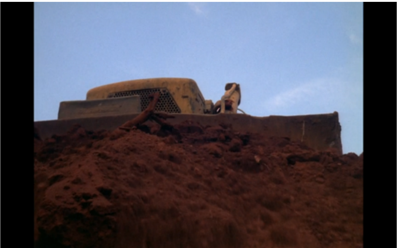
Image 4 - Bulldozer shovelling dirt as if to bury the camera.
