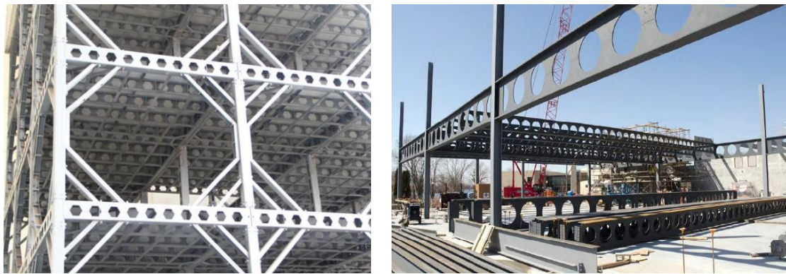
Figure 1.4 Castellated and cellular beams used in constructional industry
