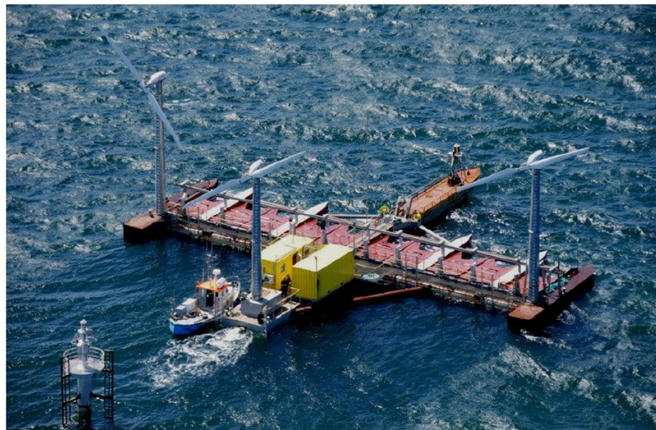
Figure 7. Poseidon hybrid wind–wave energy platform, developed by Floating Power Plant. Image taken from Ref. [44] “McTiernan, K.L.; Sharman, K.T. Review of Hybrid Offshore Wind and Wave Energy Systems. J. Phys. Conf. Ser. 2020 , 1452 , 012016.” Copyright 2020 Author(s), licensed under a Creative Commons Attribution (CC BY 3.0) license.
