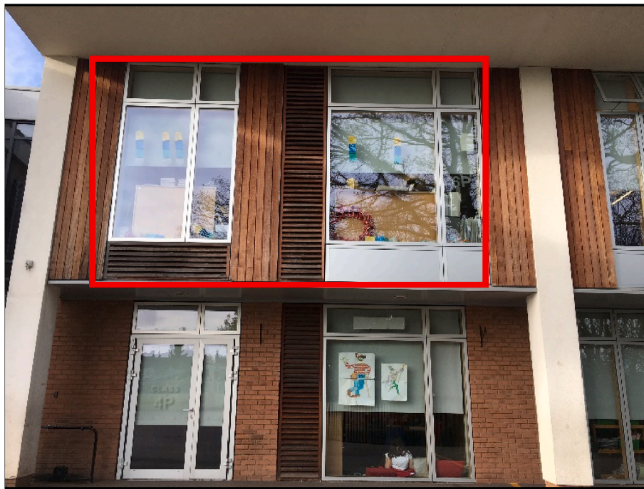
Fig. 11. A classroom in school 6 providing louvre openings alongside windows.
