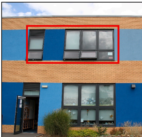
Fig. 10. A classroom in school 1 providing louvre openings alongside windows.
