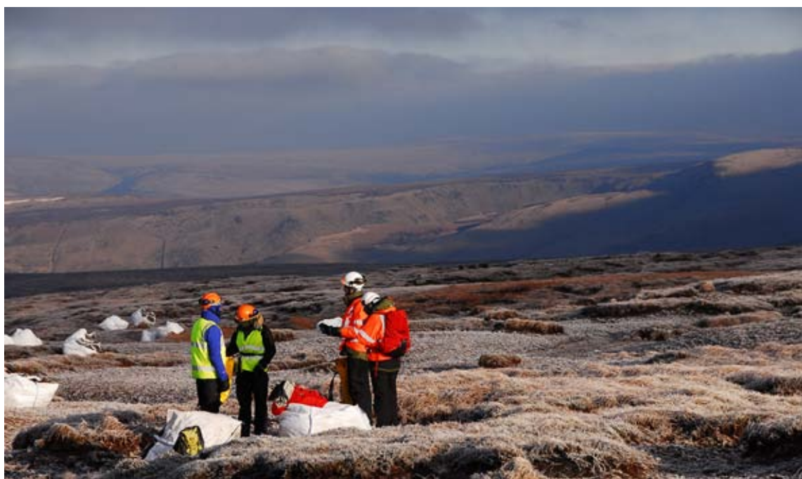
Restoration at Kinder Edge © Moors for the Future
