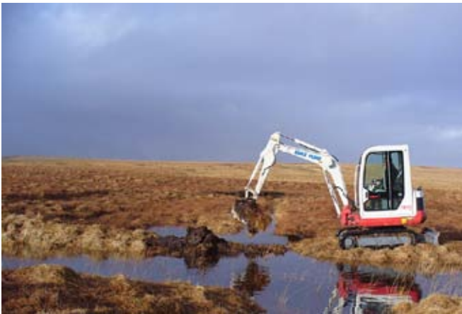
Restoration at Blackpitts © Exmoor National Park Authority
