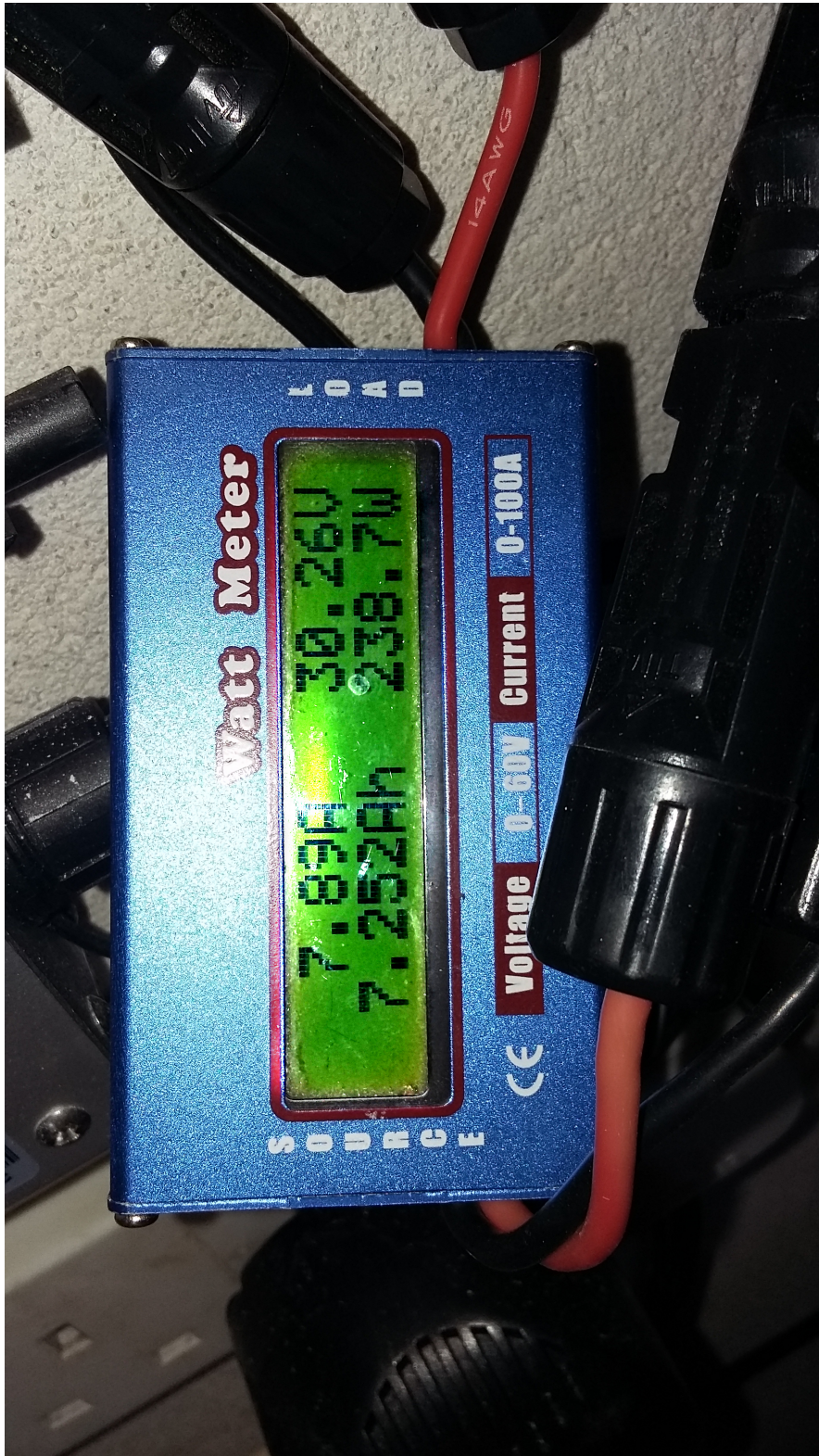
Fig. .59: Non-constant output voltage prototype assembly power measurements from testing
