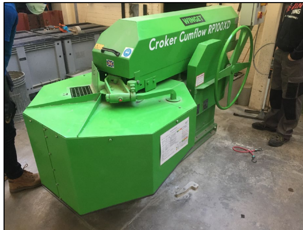
Figure 15: Concrete being mixed
