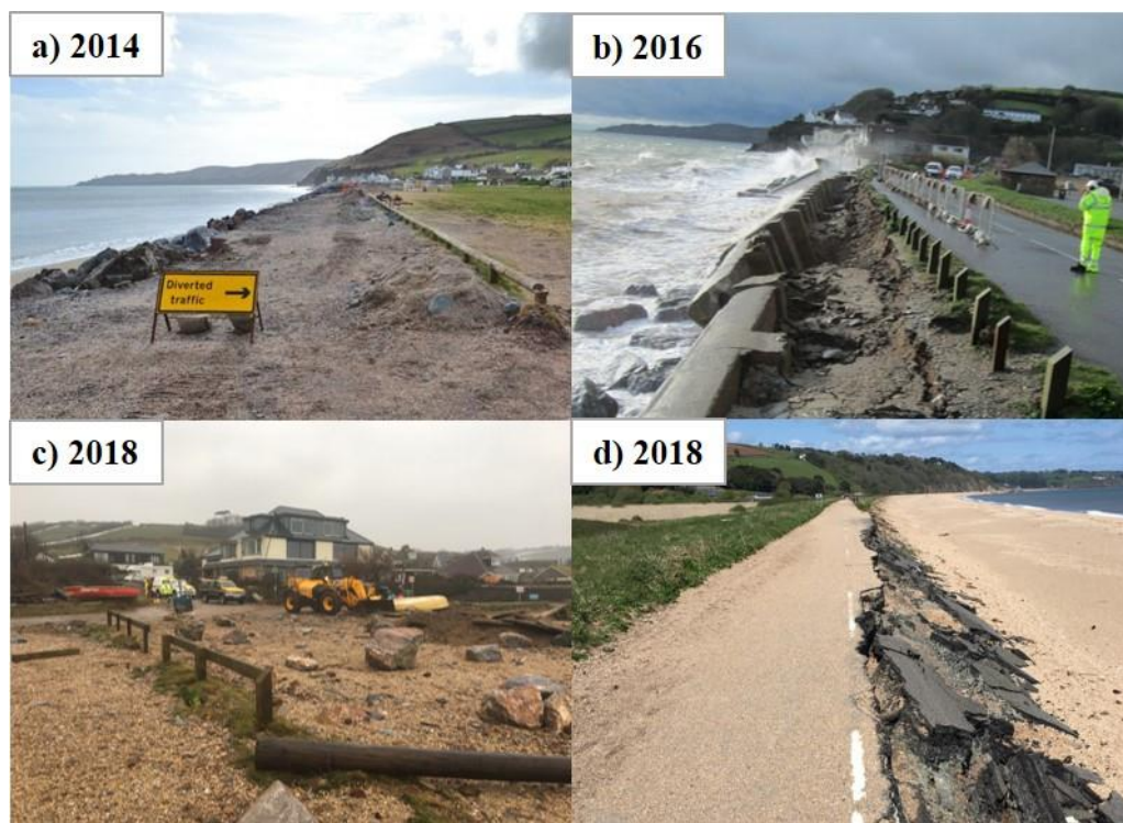
Figure 1.10. Contemporary storm damage issues in Start Bay a) Road destruction at Beesands following southerly waves brought in by Storm Petra, February 2014, b) undermining and collapse of sea wall at Torcross, Slapton Sands following sustained southerly incident waves and lowest recorded beach levels in February 2016, c) evacuation of residents following high tide impact of Storm Emma, March 2018, d) the second collapse of the A379 road atop the Slapton Sands barrier ridge following Storm Emma, March 2018.
