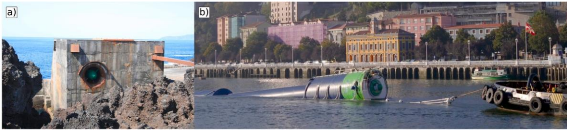
Fig. 1. (a) Shoreline OWC power plant equipped with a Wells turbine at Pico island, Azores, Portugal. (b) The IDOM Marmok-A-5 spar-buoy OWC equipped with a biradial turbine being towed for deployment at BiMEP test site, Basque Country, Spain.
