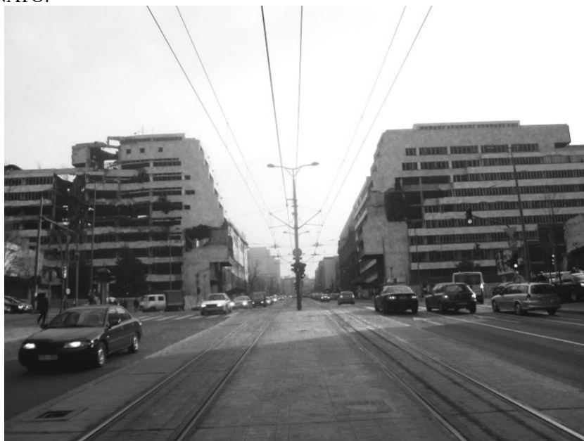
Figure 2.5 The fileted Generalstab complex in 2010, with the Military Headquarters (Building A) on the left-hand side incurring greater damage than the Ministry of Defence (Building B).
