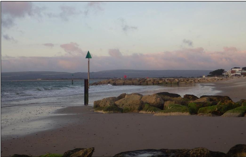
Figure 2-2. Example of an “unconnected” groyne that becomes exposed at low water (foreground) compared to a “connected” groyne that retains a constant connection with the sea even at low water (background).
