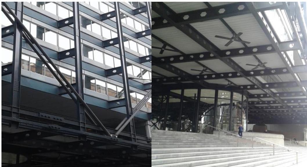
Figure 1-1 Images of application examples of castellated beams in building construction in Exchange House in London
