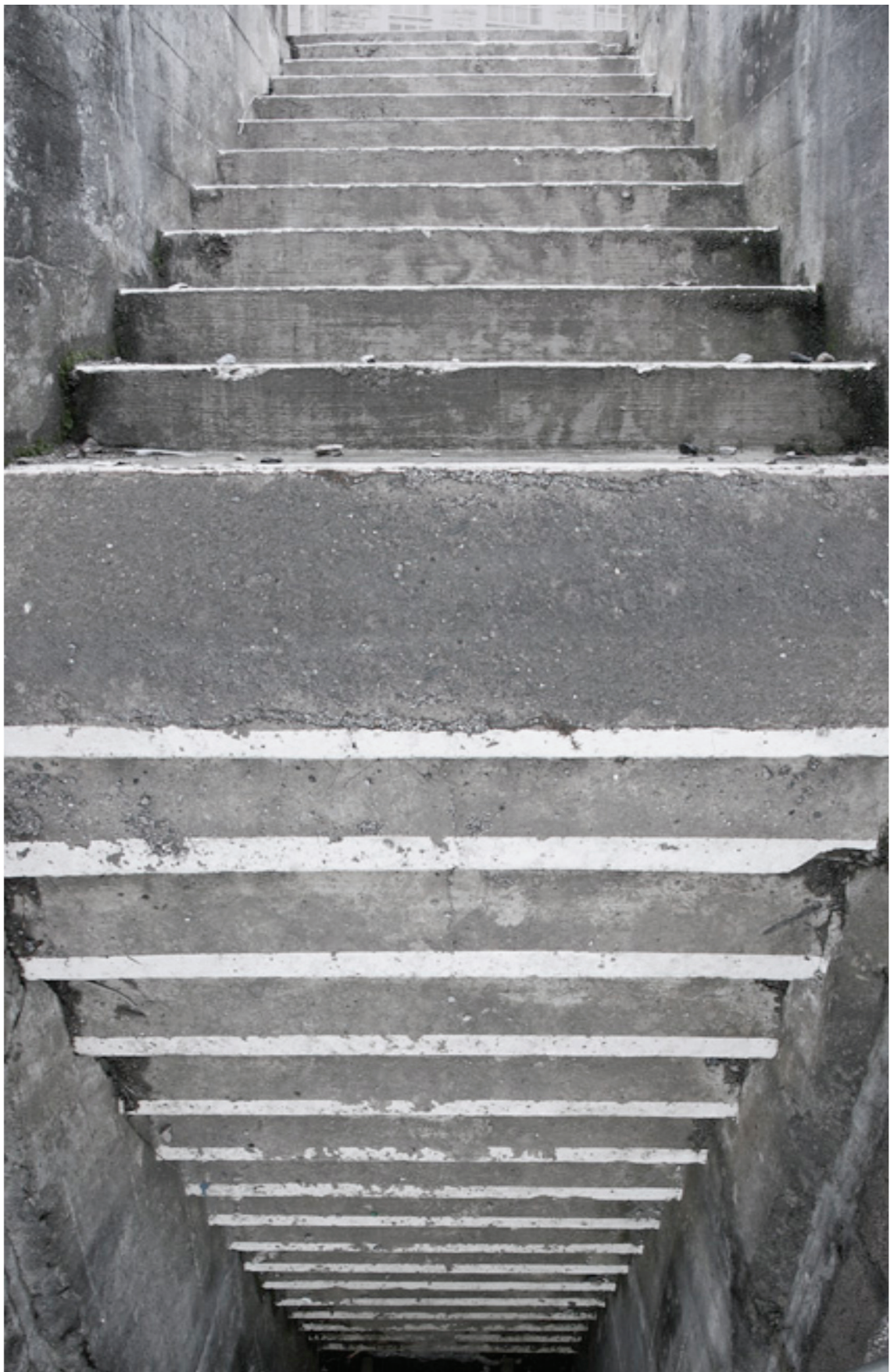
Figure 30-3. ARP bunker exit panorama
