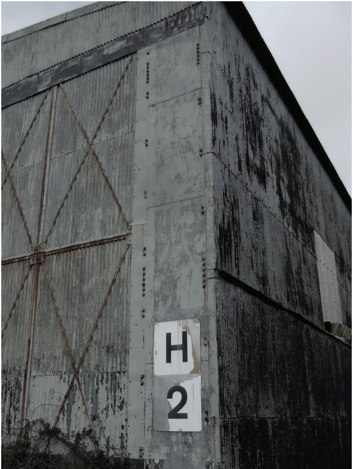
Figure 13-4. Type T2 B24 Liberator Hangar, H2
