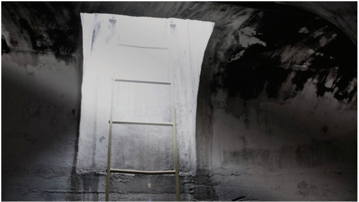
Figure 12-3. ARP bunker escape hatch
