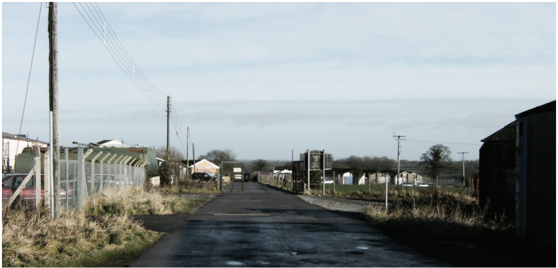
Figure 1-4. Dunkeswell airfield, Devon: access road
