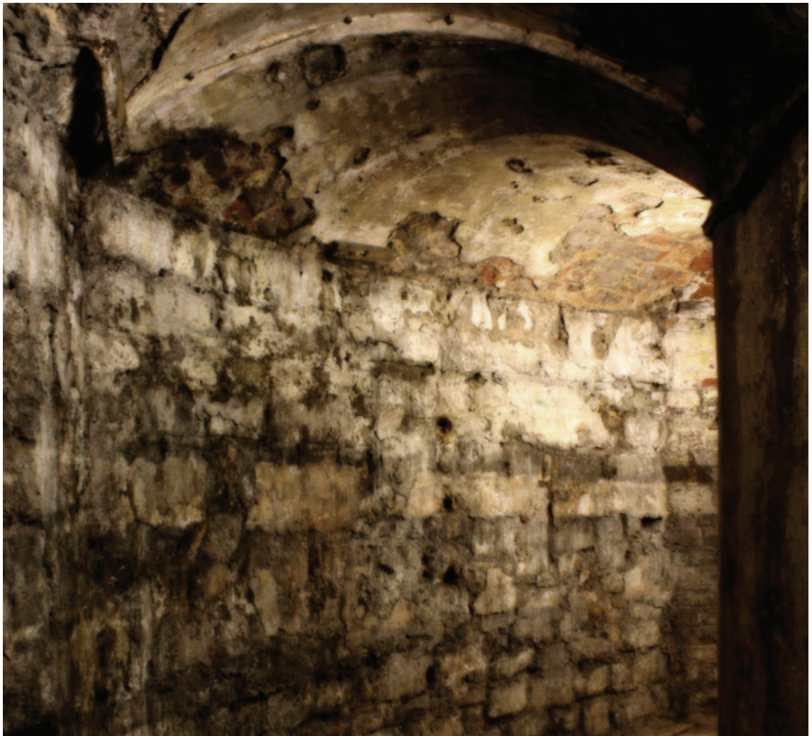
Figure 2-5. The tunnels leading to the Bath Vault
