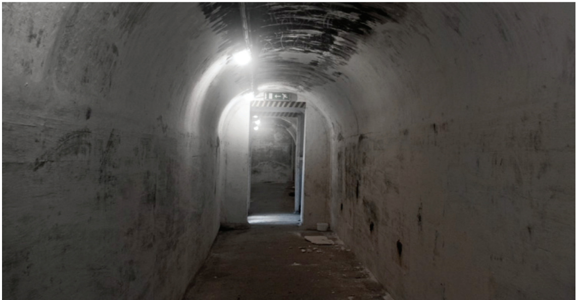
Figure 5-3. ARP bunker internal passageway
