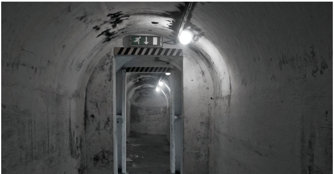
Figure 6-3. ARP bunker counterblast layout
