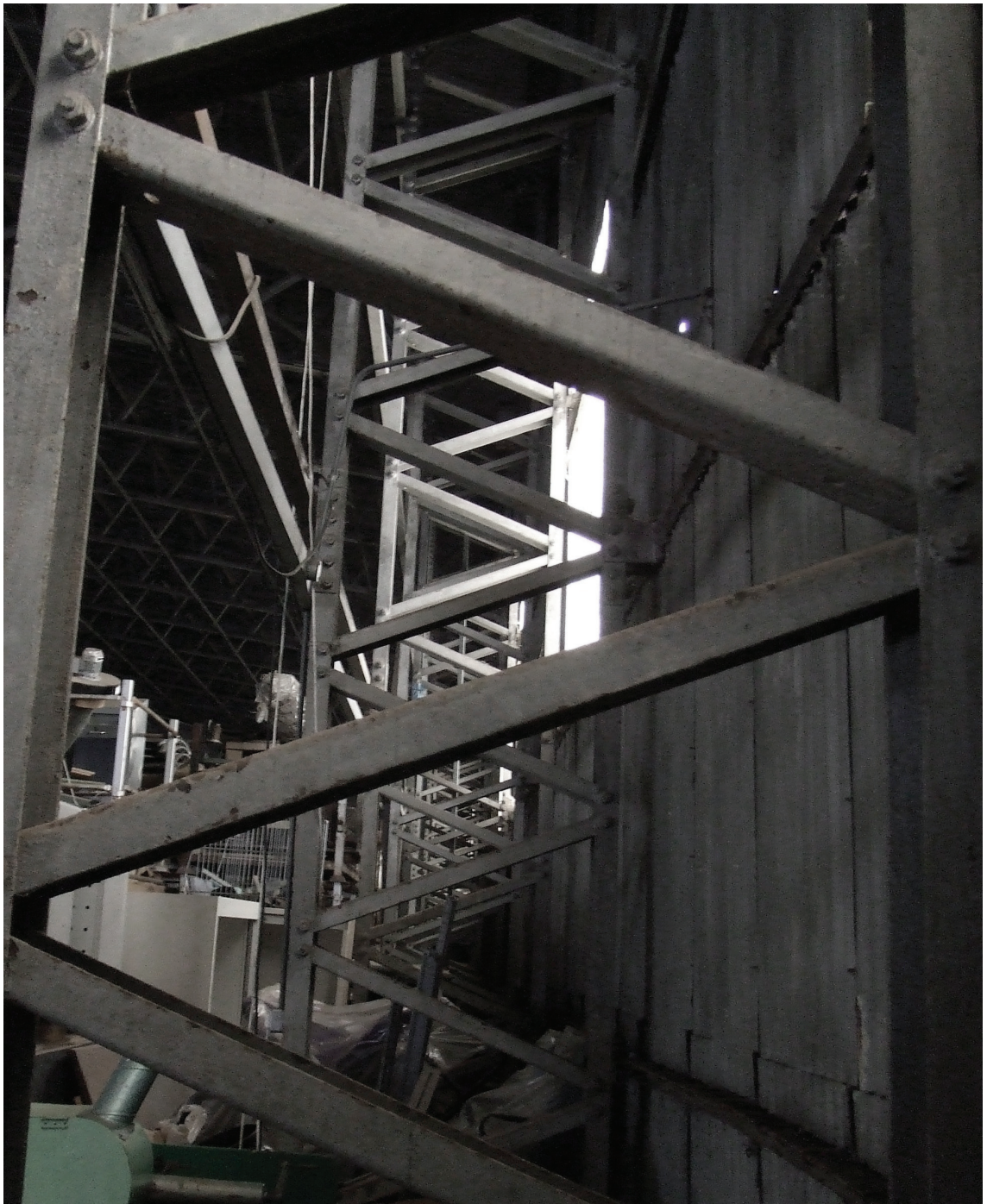
Figure 16-4. Lattice Portal Frame of Type T2 Hangar, Dunkeswell
