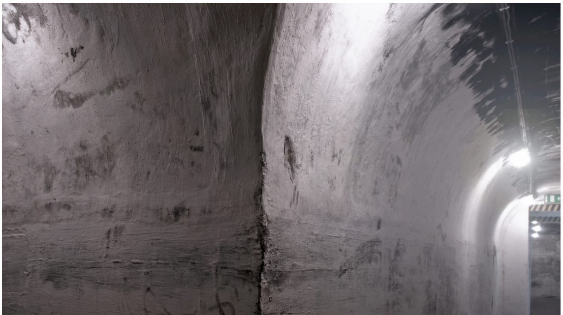
Figure 13-3. ARP bunker corner detail
