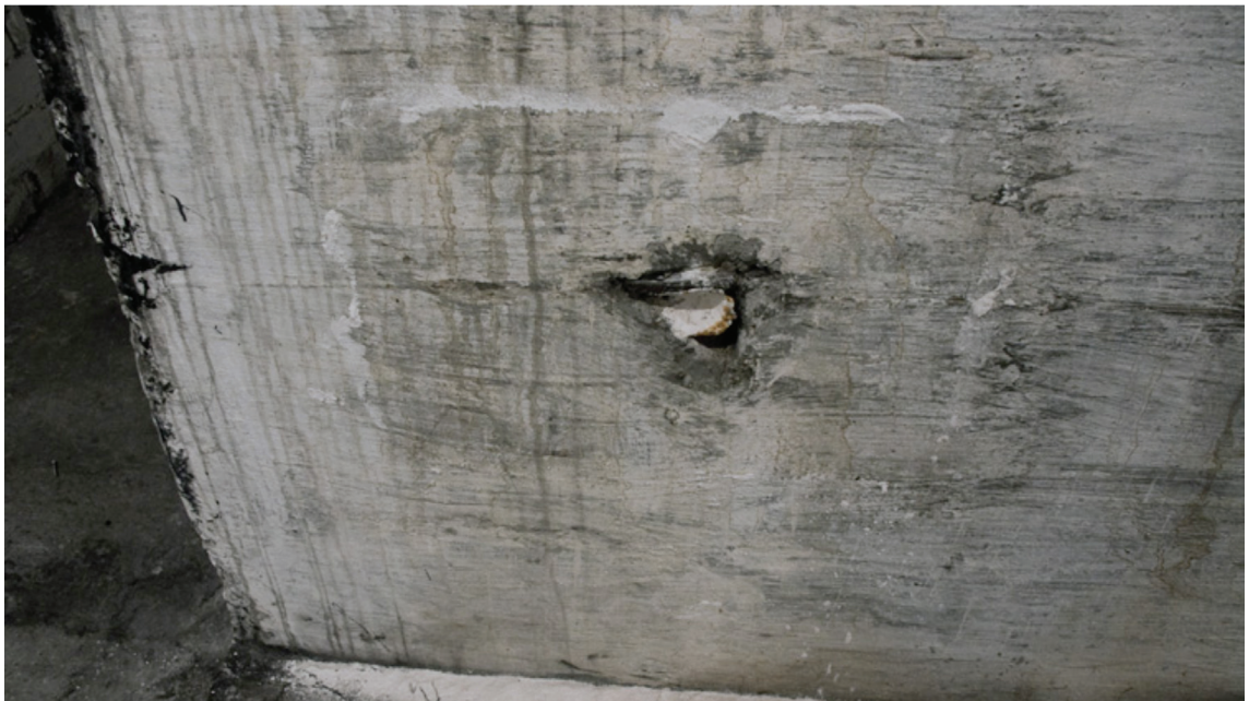
Figure 8-3. ARP bunker seat-fixing scar
