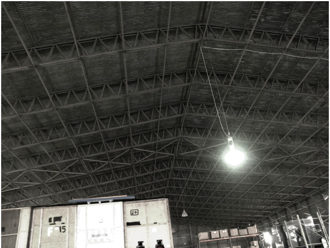
Figure 17-4. Lattice Portal Frame, roof structure: Type T2 Hangar, Dunkeswell
