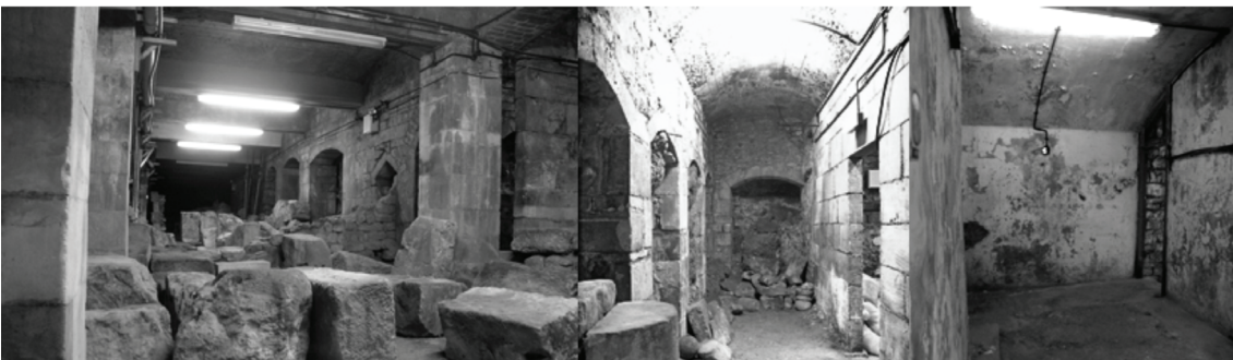
Figure 5-1. Case study 3: The Vaults, Bath
