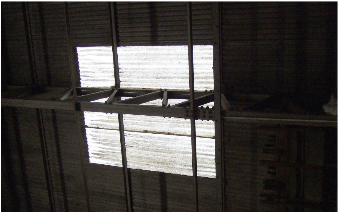
Figure 18-4. Roof span: Type T2 Hangar, Dunkeswell
