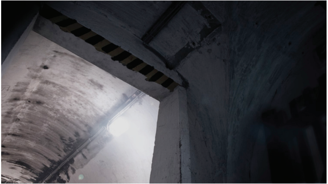
Figure 7-3. ARP bunker internal threshold
