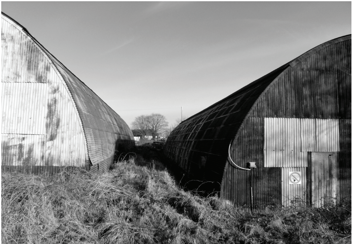
Figure 3-4. Hangars, Dunkeswell airfield
