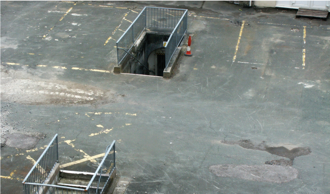
Figure 3-1. Case study 1: ARP bunker, Plymouth
