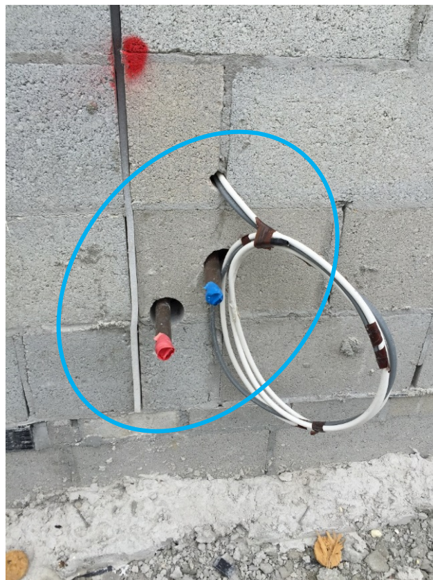
Figure 4-44 Missing insulation around pipes in Case study 5 (Source: Taken by this thesis' author)
