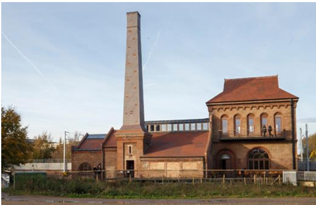
Figure 6.3 Swift holes built into renovated chimney (Source: Walthamstow Wetlands)
