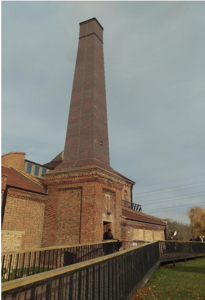
Figure 5.7 Refurbished Marine Engine House with 'swift tower' installation, November 2017.
