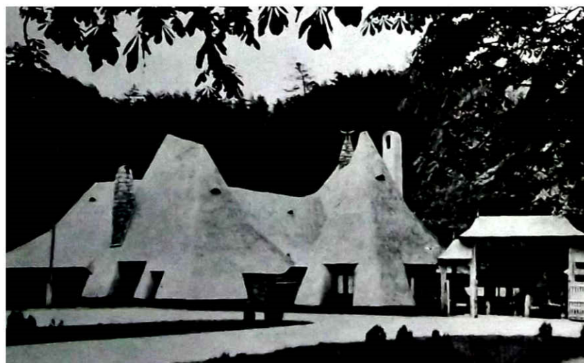
Șura Dacilor restaurant in Brașov (arch. Marian Renel, 1972).
