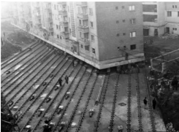
Fig. 27. Apartment building A2 (Alba Iulia) and Sfântul-Ioan-Nou Church (Bucharest) translated by Iordăchescu's team using the engineer's method (which entailed building a structural foundation 'tray' under the building, and transporting it to the new site, where the structural links between the building and a new foundation would be recast).
