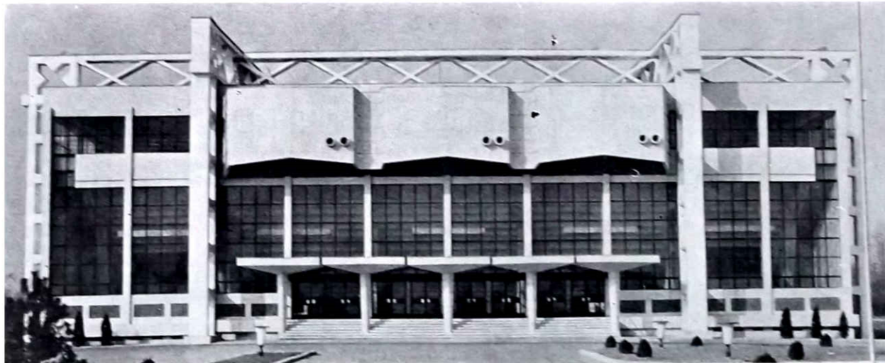
Sports hall in Ploiești (arch. Gheorghe Dumitrescu; 1968-1971).
