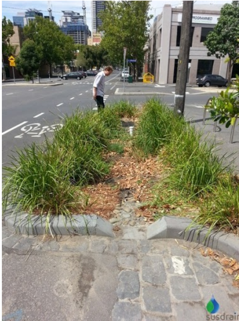
Figure 2. Bio-retention area in Melbourne (Susdrain, 2015).
