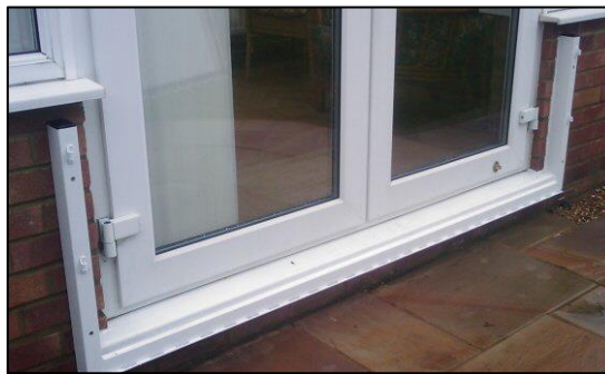
Figure 20: Barrier mount connected to the brickwork below the patio door frame (Flood Wall, n.d.)
