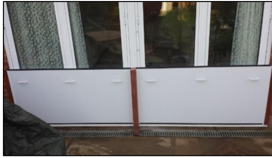
Figure 19: Barrier protecting large patio doors with a central support embedded into the ground (Stormguard, 2015)
