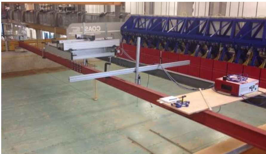
Figure 1 - Coastal Basin set up prior to filling of Basin
