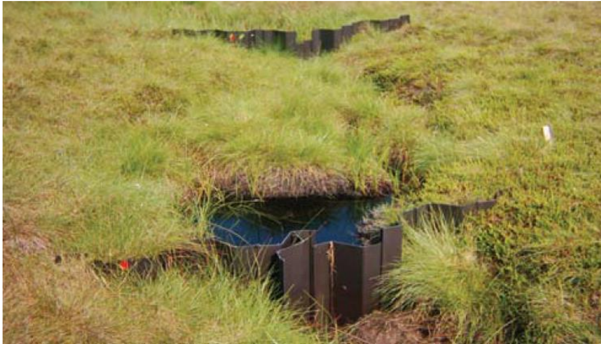
Figure 17: An example of drain blocking (Natural England, 2010).
