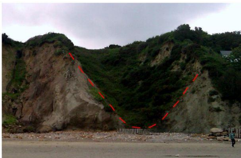
Figure 3.4 Cross-sectional shape of a Translational (planar) landslide (16) in Whitecliff Bay (south).
