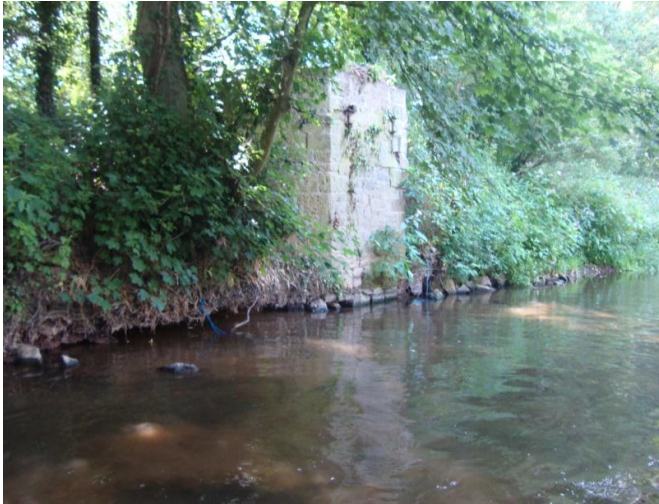
Plate 7. The blockwork foundations located upstream of Site 2 entrance that were under construction to provide a footbridge over the river.
