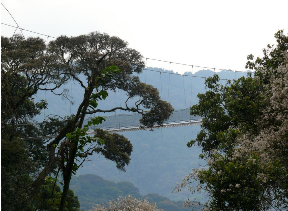
Picture 3: The Nyungwe canopy walkway in Rwanda was build by Greenheart Conservation Company Ltd. in 2010. The construction consists of three towers, three platforms and 165m of bridge connections.
