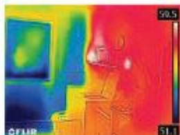
Uninsulated Outside Wall
