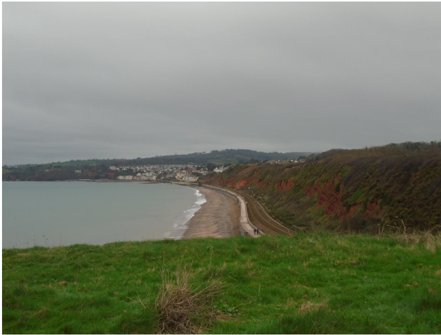
Figure 22. Top of Langstone Point, rail track below.
