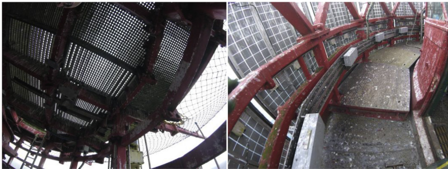
Fig. 17. Eddystone helideck views. Left: helipad, right: vertical structure rising from the gallery, with solar panels attached.
