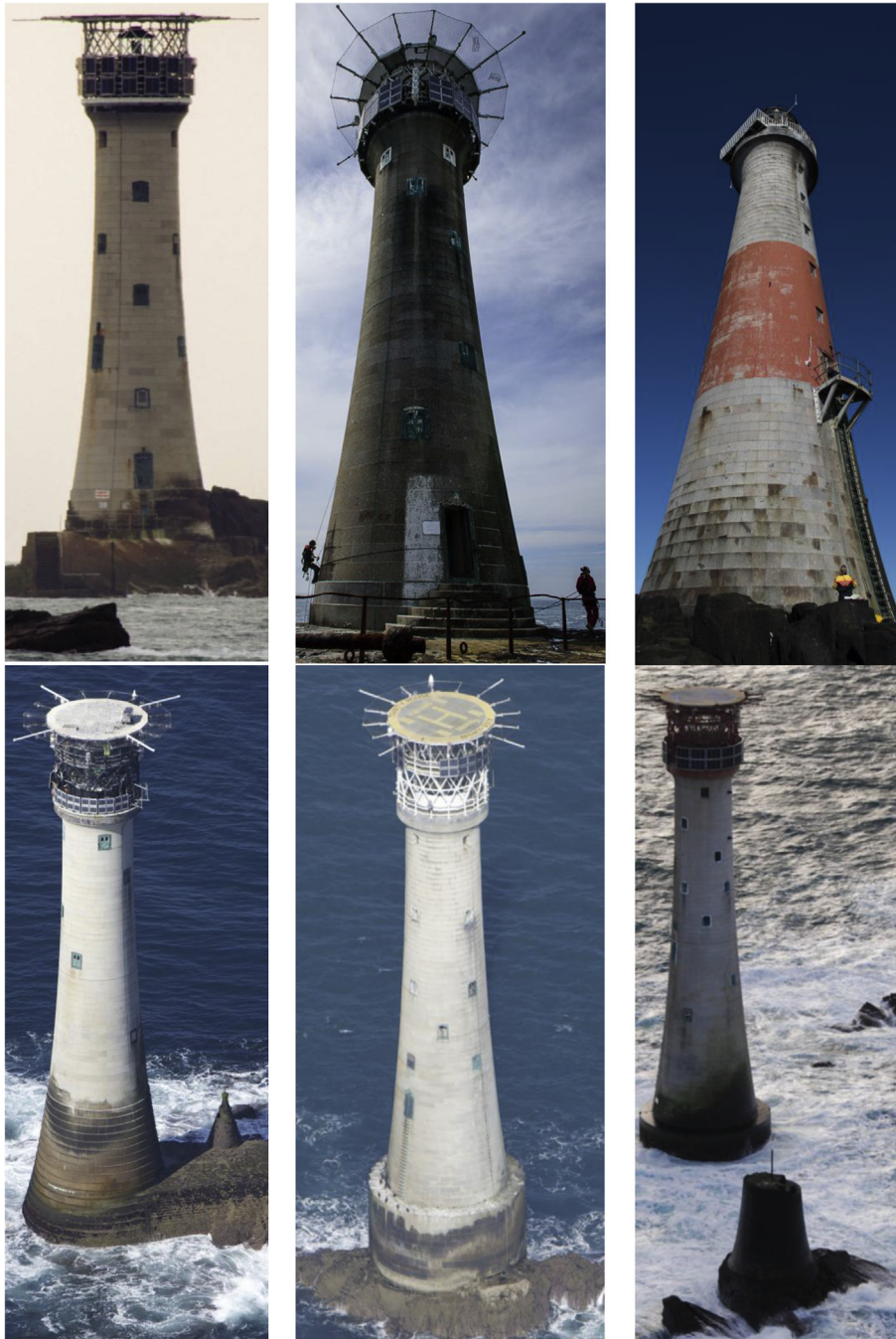
Fig. 1. Rock lighthouses around the British Isles. Upper row from left: Les Hanois, Longships, Dubh Artach (author photos). Lower row from left: Wolf Rock, Bishop Rock and Eddystone (Lower row photos courtesy of Trinity House).
