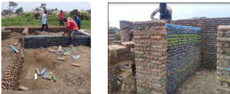
Figure 8: Plastic bottle Wall construction
