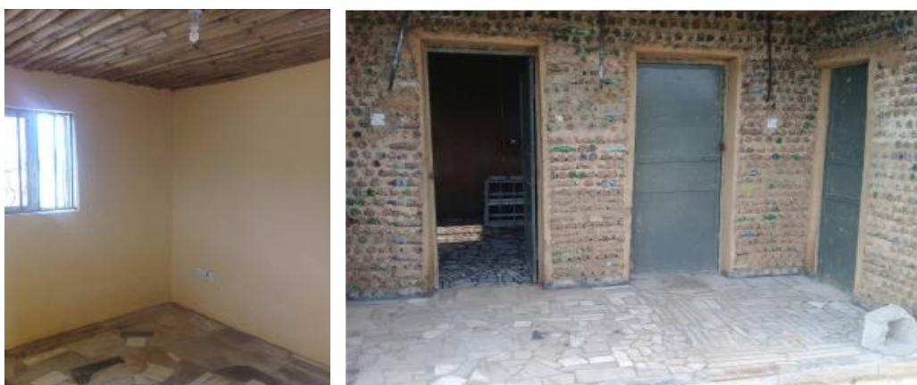
Figure 10: Plastered walls and finished floor.
