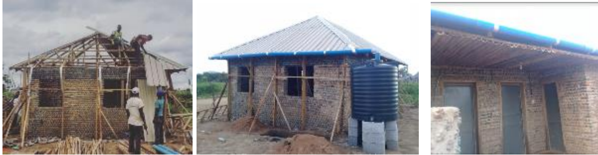
Figure 9: Roof Construction with rainwater harvesting
