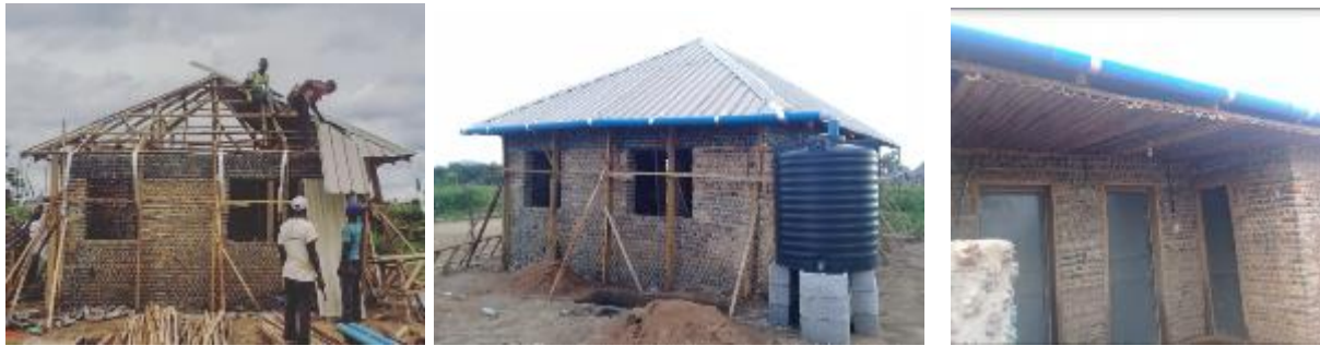
Figure 9: Roof Construction with rainwater harvesting
