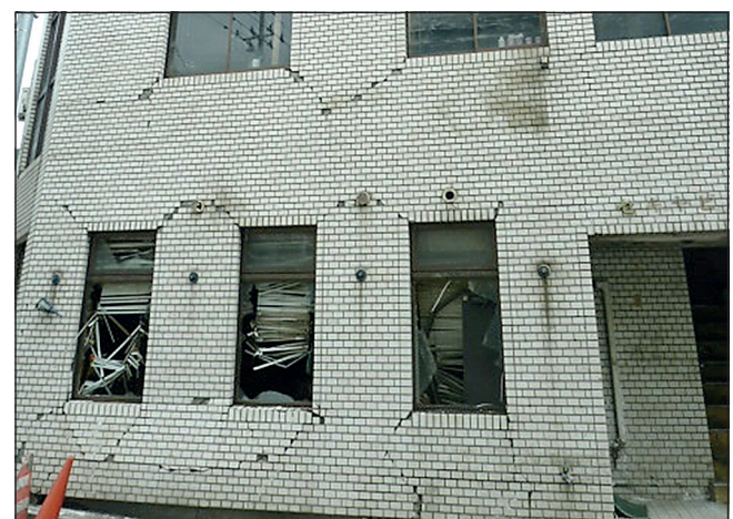
Figure 4. Tsunami-preceding seismic damage indicated by conjugate shear cracking of a building facade in Kamaishi
