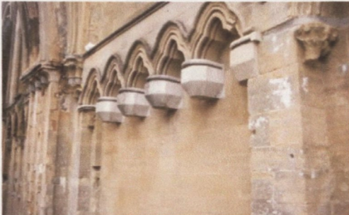
Figure 21 Glastonbury Abbey, Somerset. The honesty of the carved capitals - left as blank rough-outs - the lack of any attempt to restore historic detail - shows the influence of SPAB on the restoration versus repair debate.
