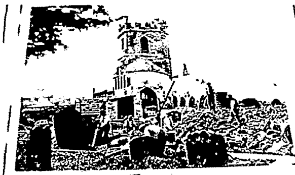
Broadwindsor Church Figure 26 Broadwindsor, Dorset, showing the chaos of a nineteenth century restoration. Note the heaps of rubble in the foreground, and the apparently surviving areas of plaster wall above the nave arcade. This survey failed to find any evidence of surviving plaster. ( On display in the church, original photographer unknown. )
