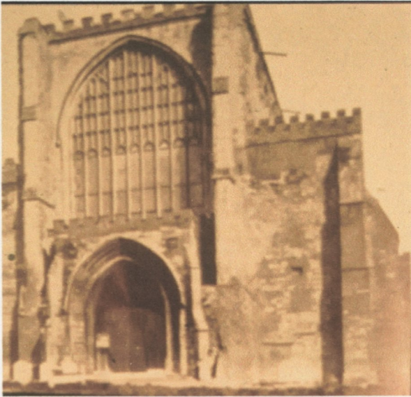
Figure 19 St. Albans Abbey, before restoration. Detail of west end.
