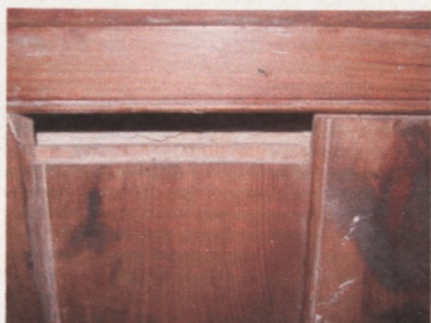
Figure 51 Warmwell. Medieval plaster protected behind wainscot.
