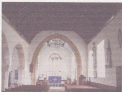
Figure 50 Winterbourne Martin. Neatness and regularity in the layout of fittings, typical of through Victorian re-ordering.
