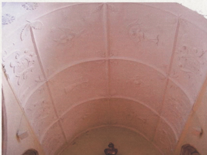
Figure 27 Abbotsbury, Dorset : Hand modelled plaster ceiling.
