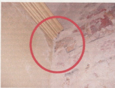
Figure 45 Puncknowle, junction of the north arcade wall with the chancel arch, showing the complex relationship of plaster fragments
