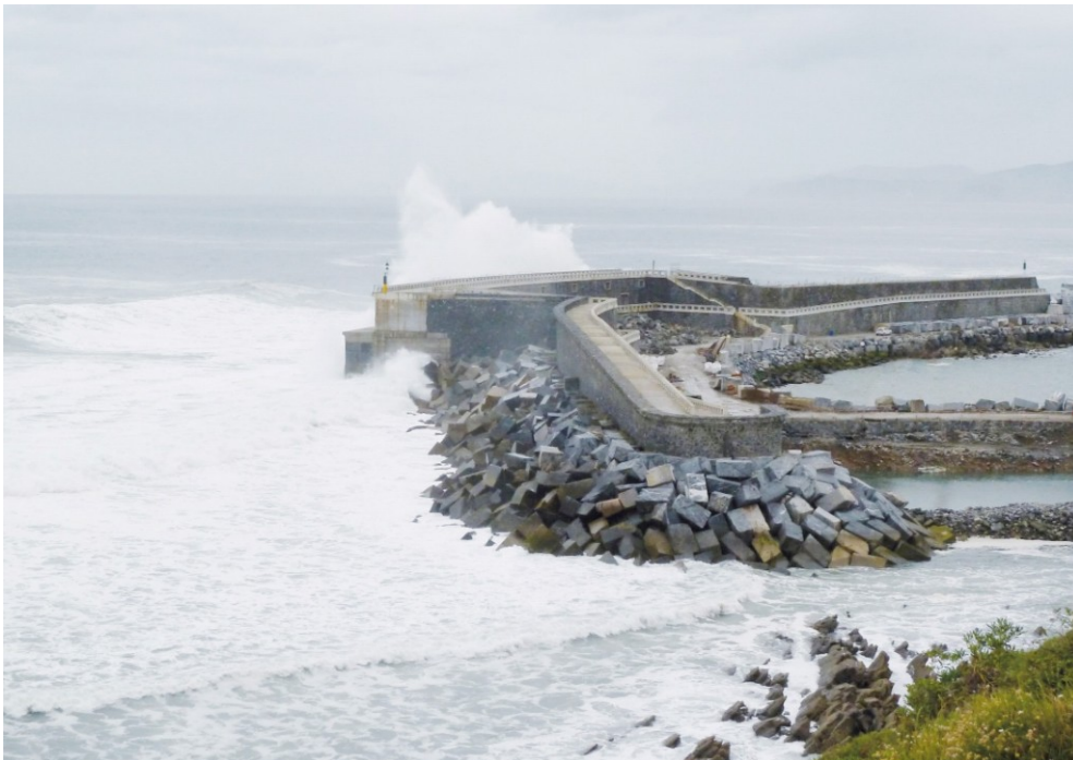
Figure 10: Mutriku breakwater view.
