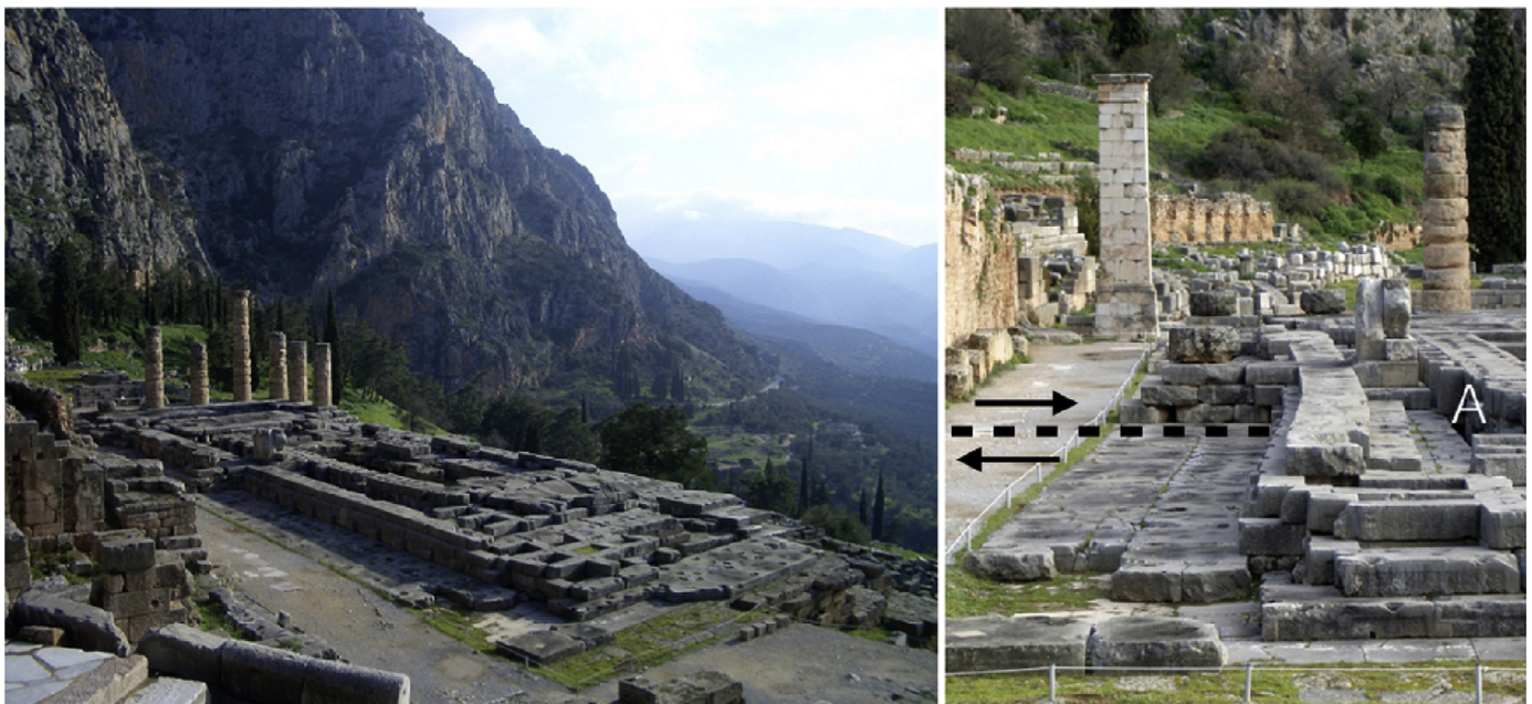
Fig. 10. (a) General view of the Temple of Apollo at Delphi, and (b) a close-up showing its inner walls markedly bent at its intersection with the trace of the inferred cross-fault. The implication is that the oracular chamber below the temple complex lies on a line of minor fault movement.
