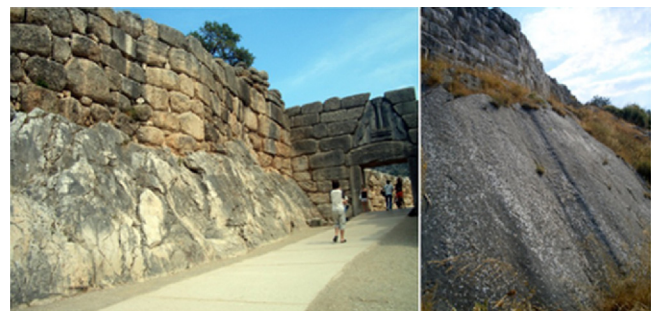
Fig. 2. The formidable 'Cyclopean Walls' of the hilltop citadel of Mycenae are built atop metre-high limestone fault scarps, with the southeastern one bordering the famed Lion's Gate entrance (a) and the northeastern one that lies along the line of the sacred Spring (b).
