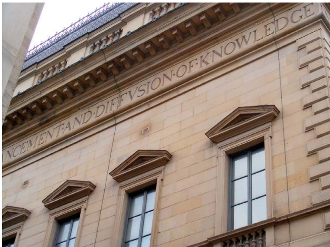
Figure 14. Manchester Athenaeum, designed by Charles Barry, built 1824-1835. Author's photograph, 2010.
