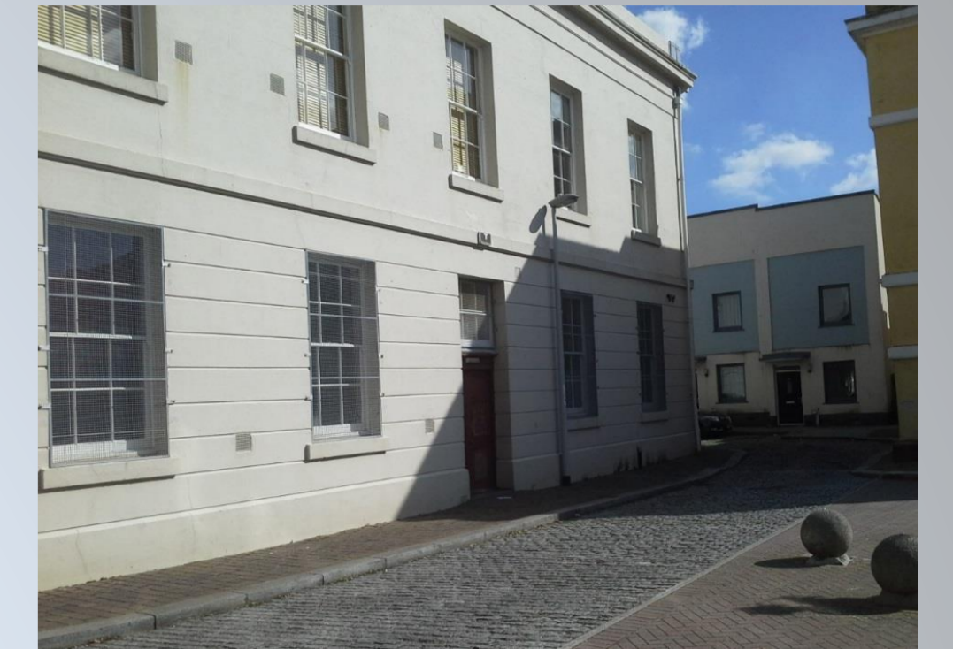
Ker Street Police Station
