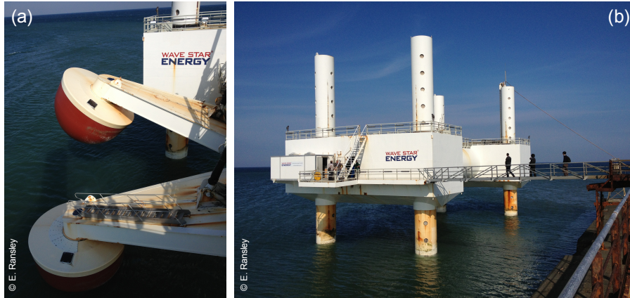
Figure 1: Photographs of the Wavestar prototype near Hanstholm, on the west coast of Denmark. Showing 2 point-absorbing floaters (a) and the supporting platform and 4 monopile foundations (b). Photo Credit: E. Ransley (Sept. 2013).
