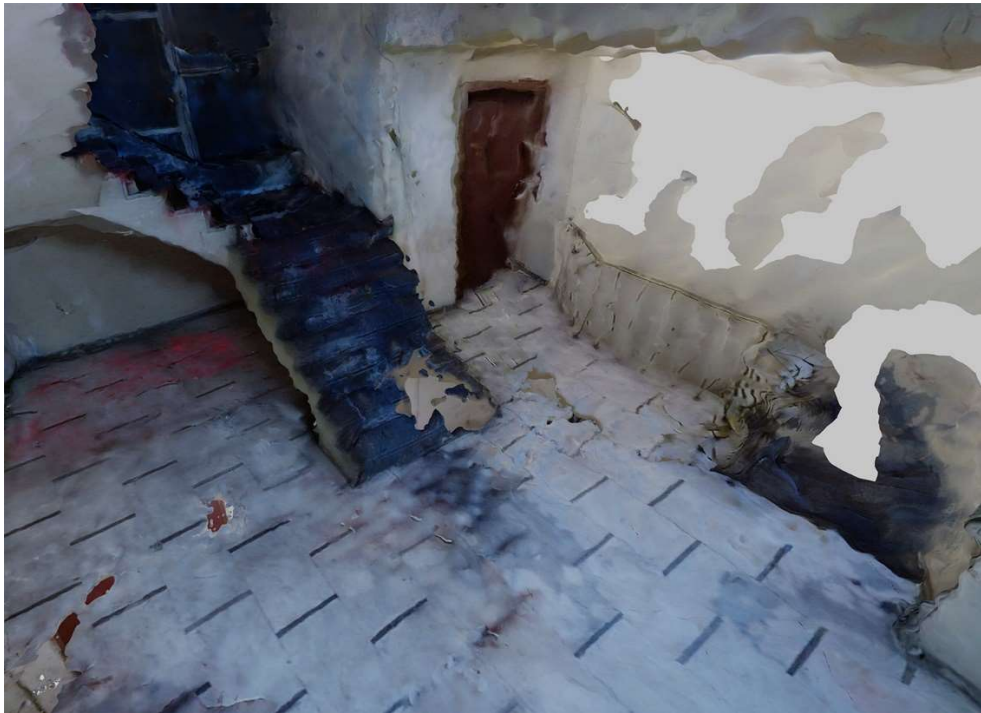
Figure 30. Polykatoikia stairs A
