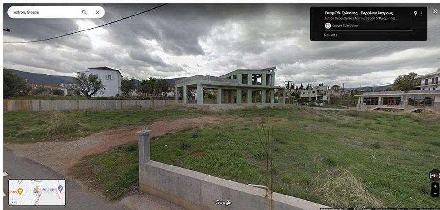
Figure 60. Yapi , Google Street View, November 2011 (©2023 Google)
