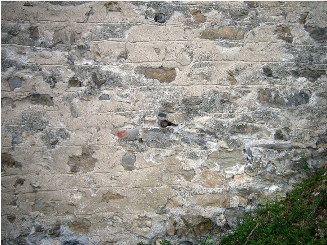
Figure 66: Outside wall of the ruin Ruchenberg: Pietra Rasa with grout marks
