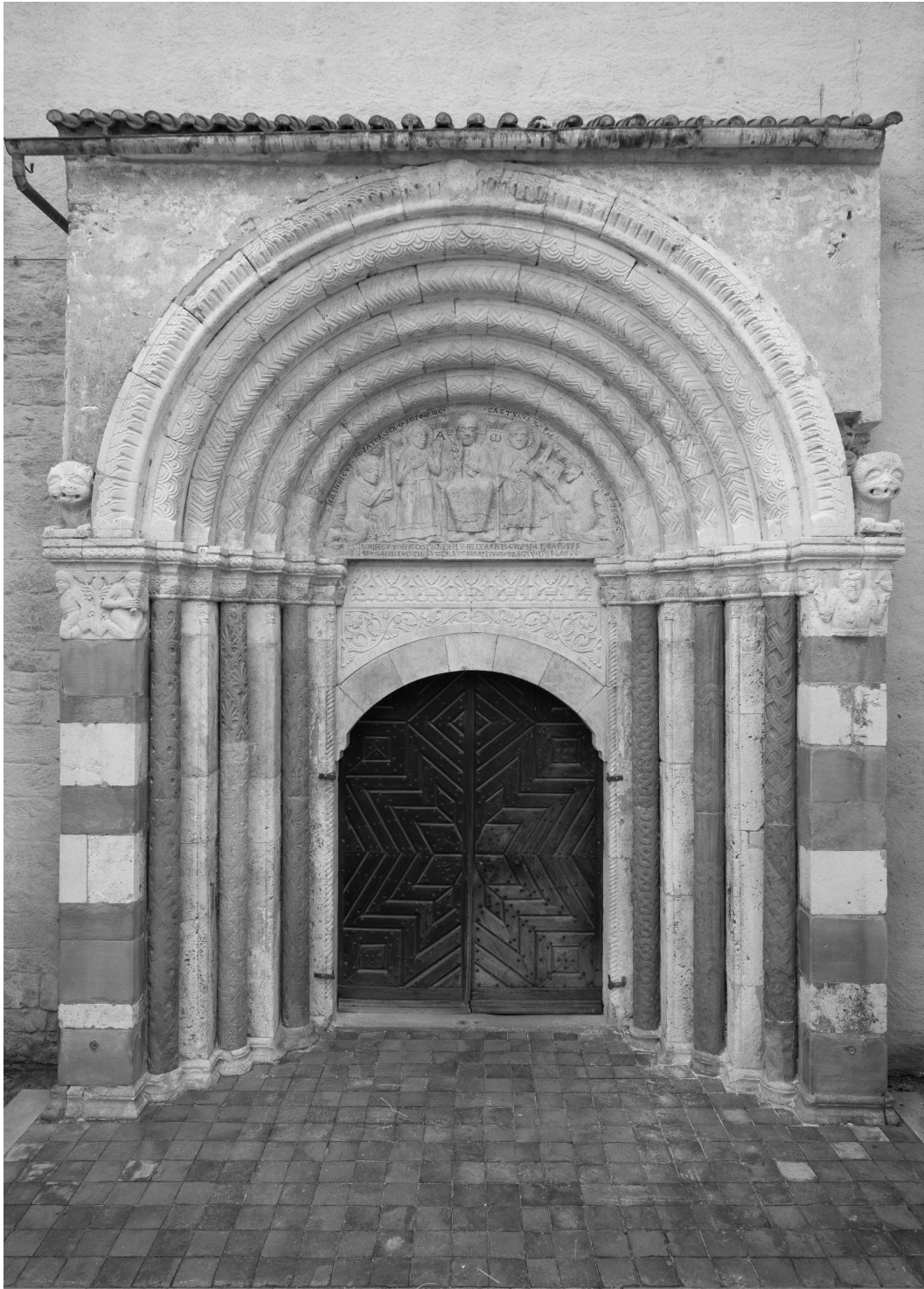
Figure 47: Photography of the portal
