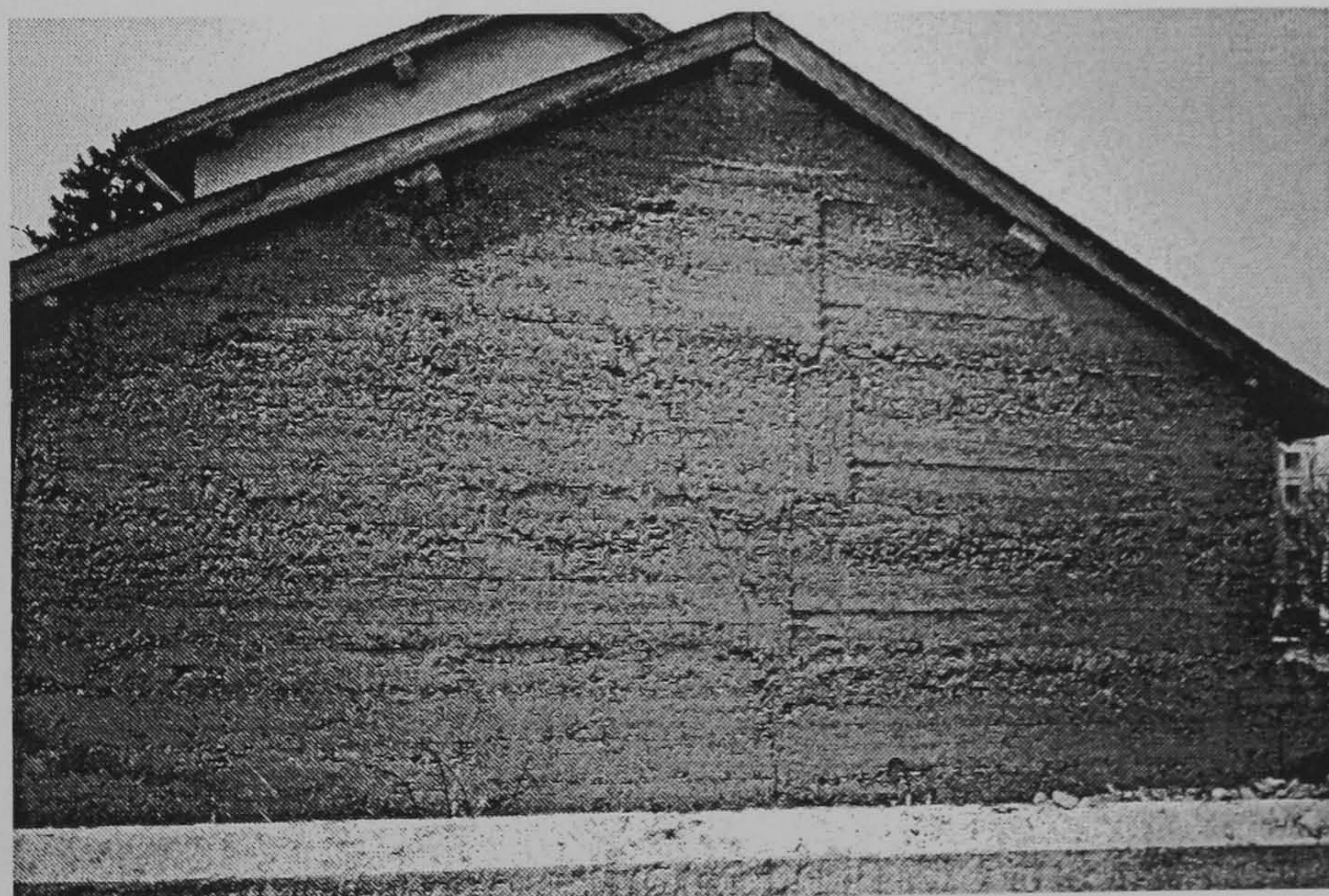
Figure 1.3 French rammed earth, ' pise de terre ', (single storey dwelling).
