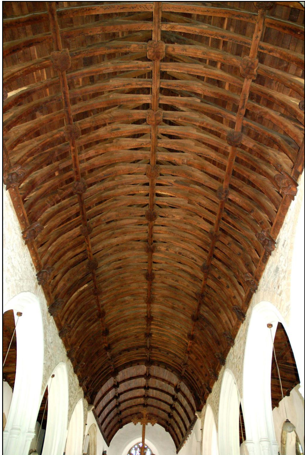
Fig. 6.16 South Tawton nave and chancel roofs.
