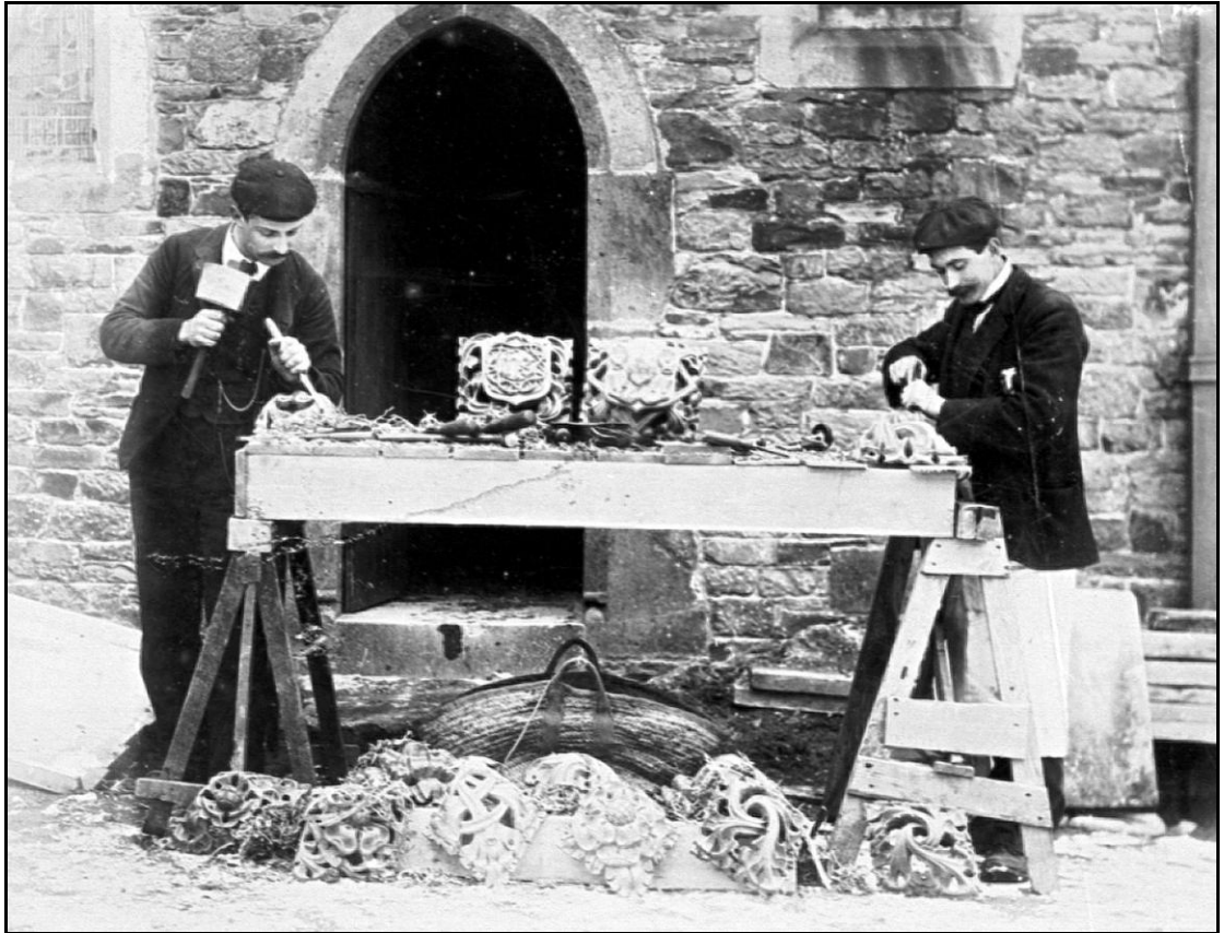
Fig. 2.25 Carvers at work on roof bosses outside Winkleigh church, c.1900. Photograph by Edward Saunders (?).
