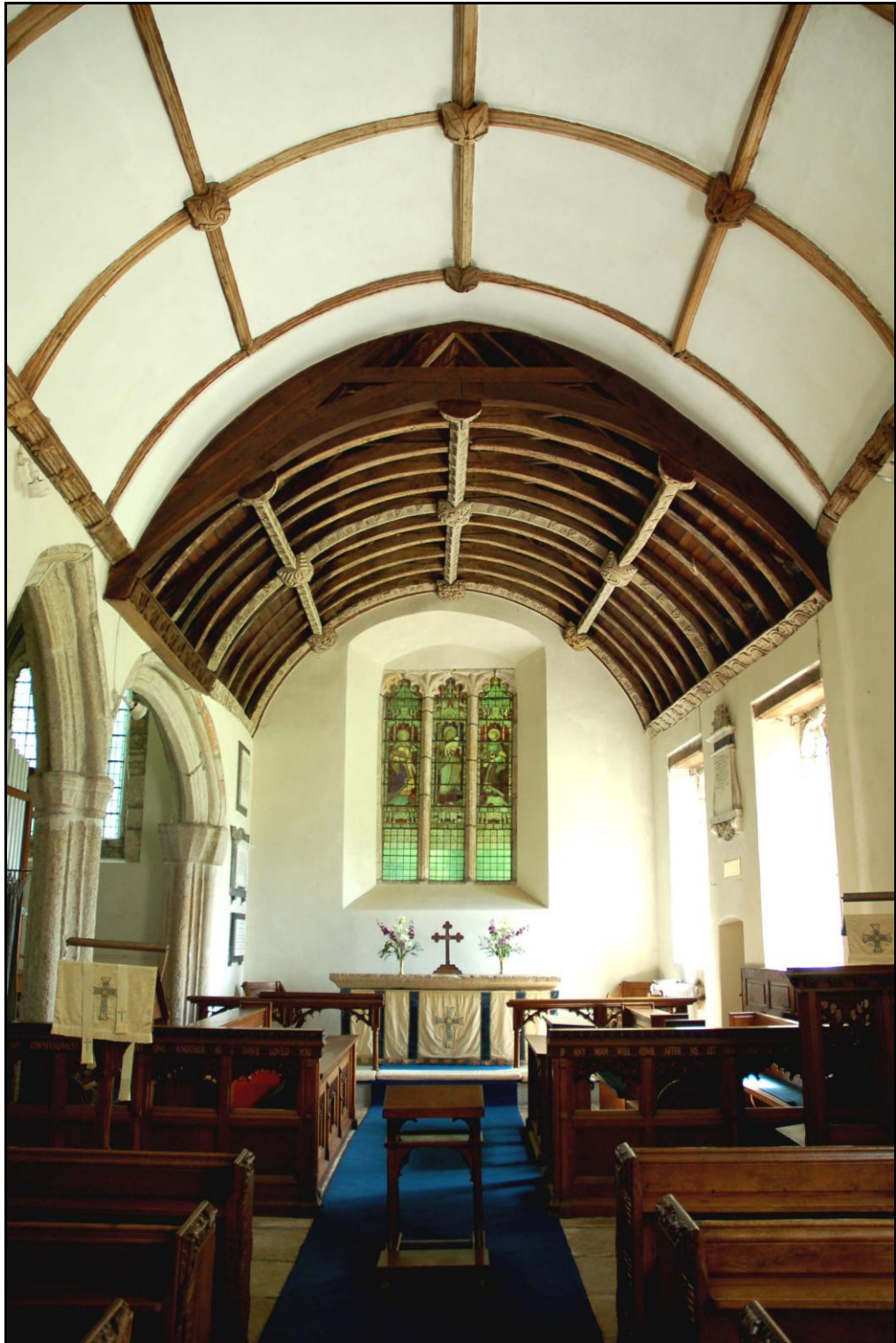
Fig. 6.6 Spreyton chancel and nave roofs, 1451.
