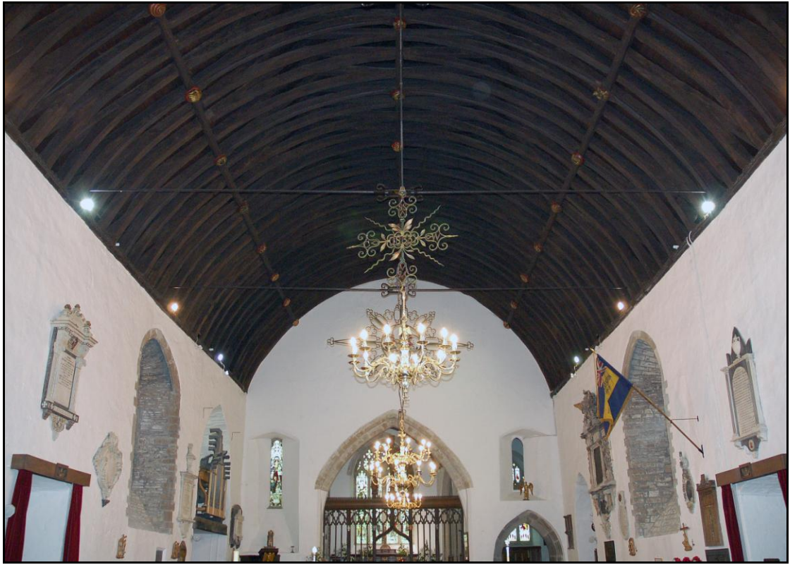
Fig. 6.4 Braunton nave roof, c.1388–1413.
