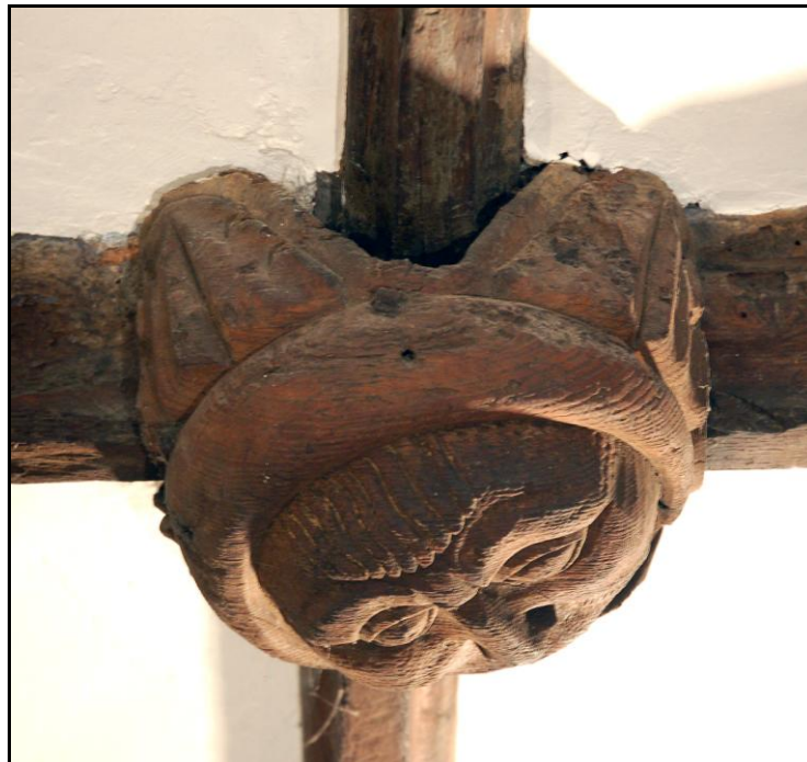
Fig. 2.21 Head, roof boss carved with 'wings' reaching up into the angles between ribs and purlins, North Molton nave, 15 th C.
