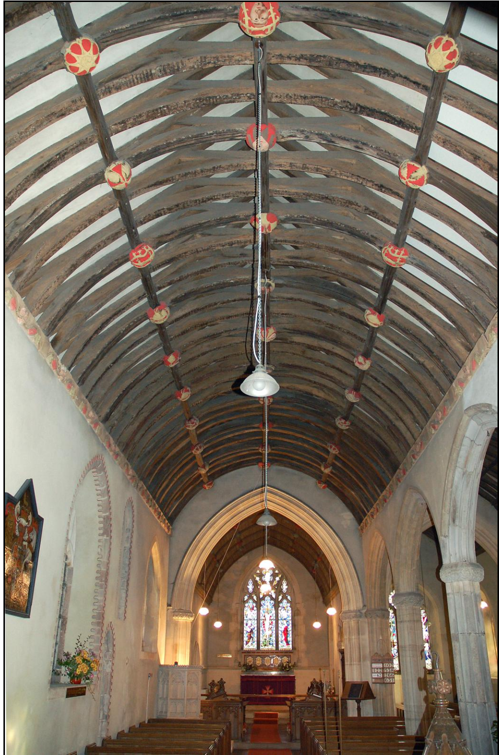
Fig. 6.1 Stoodleigh nave roof showing 30 of 33 roof bosses.
