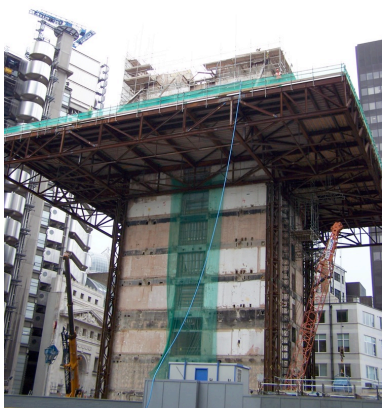
Figure 5. Tower construction site, And While London Burns (2006)
